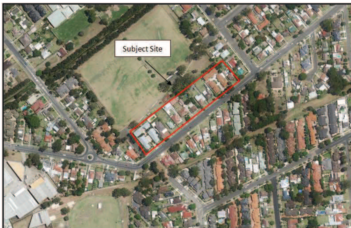
Figure 1: Aerial photograph of subject site
